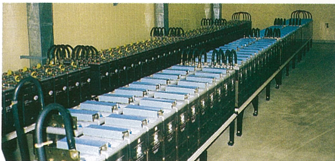
The battery bank at Itaipu provides 2 million Ah of backup capacity
