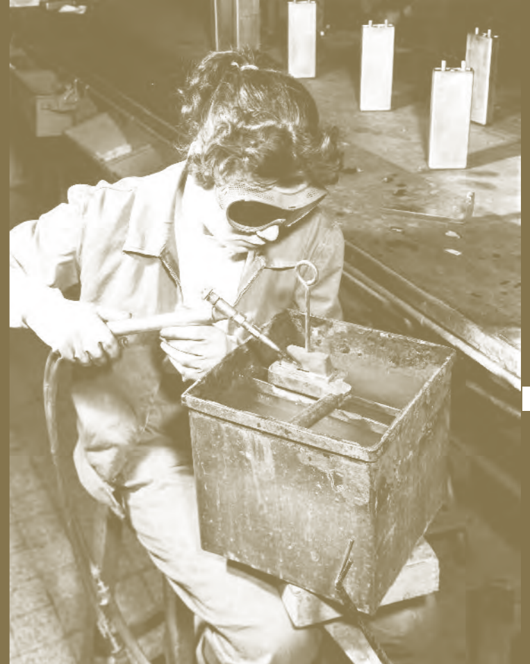
Battery casing welding
