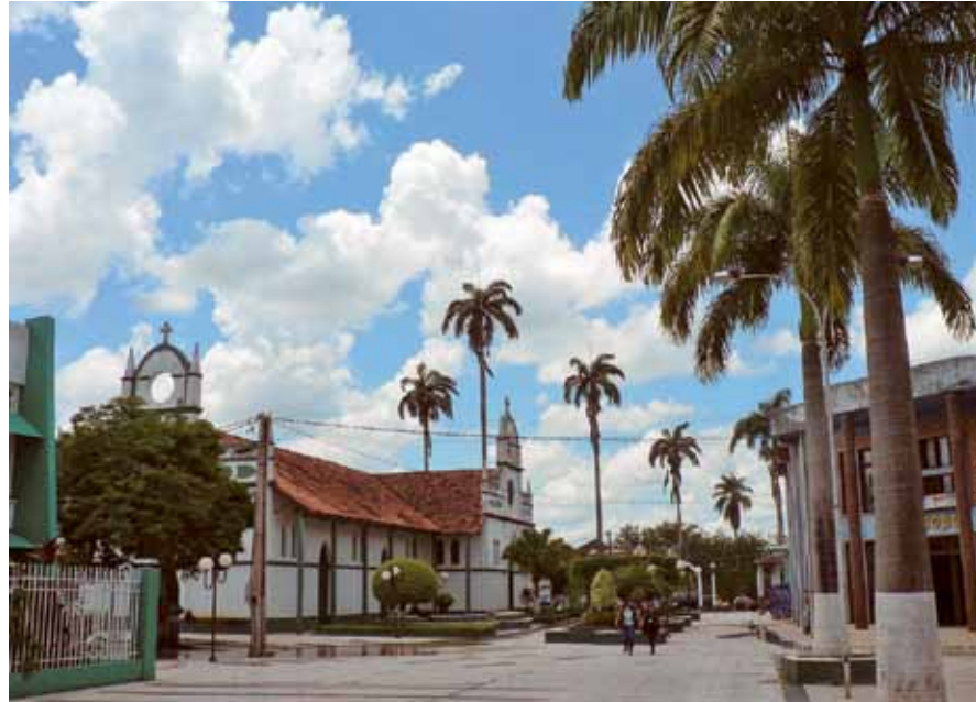
Cobija, Pando's capital. Pando is not connected to the country's national grid, resulting in electricity coverage of just 65%
